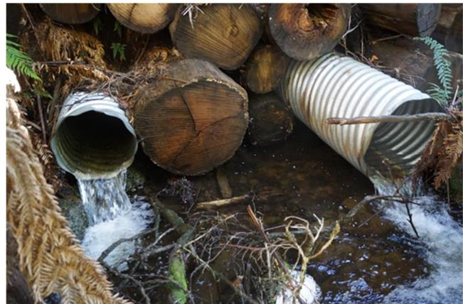
Figure 5-3. Temporary log crossing in use as a forwarding track across a permanent stream in tall, wet eucalypt forests in Victorian Central Highlands region. Source: Jacobs (2020).
