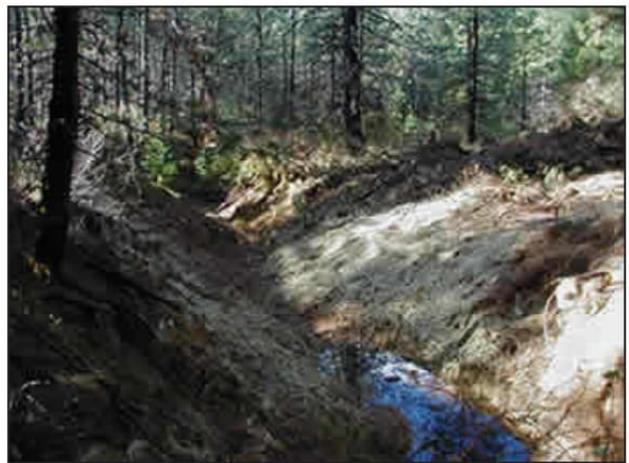
The situation was an ephemeral drainage line used during August, when the chance of measurable precipitation was minimal. The crossing was removed by September 1. There was no pipe or separator material used. Whole trees 250-600mm diameter breast height were used in the drainage channel. After the crossing was no longer needed, the material was removed with a heel-boom loader and processed at the landing. Standard erosion control measures were required.
